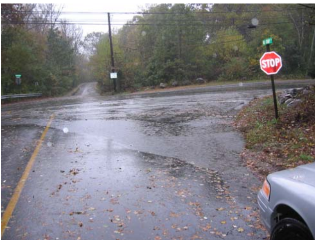
Trapelo Road at Old County Road
